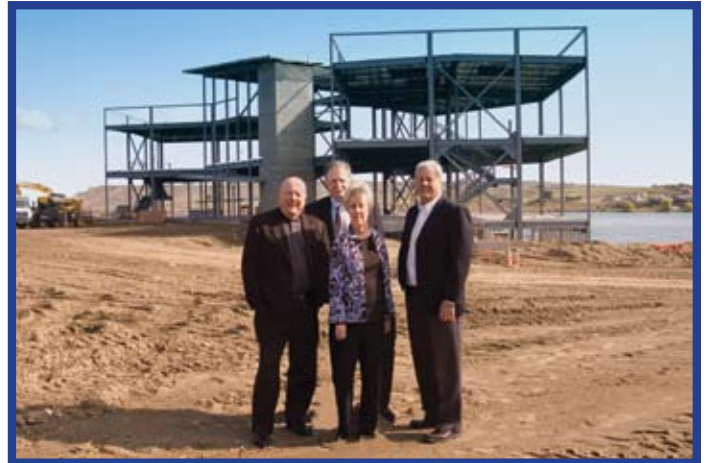
Dick French, Jim Watts, Lucy Love and Bill Lampson are standing in front of their new construction project, an office building overlooking the Columbia River and Hanford Reach.
