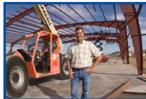
Jim Early inspects new warehouse building.
